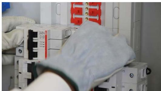
The Breaker Snaps Into The DIN Rail
